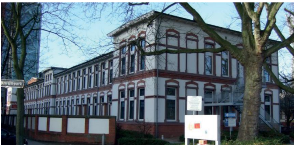
The ZfAM in house 1 of the St. Pauli Health Centre, formerly known as the harbour hospital 141
